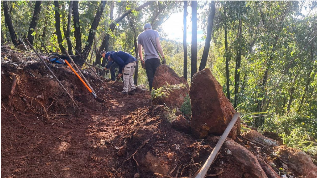
Figure 9 Mountain Bike Club members constructing track in Glenwood State Forest. (photo obtained from Club Facebook page). Note the wide area of disturbance, deep cut, exposed roots and displaced boulders.
