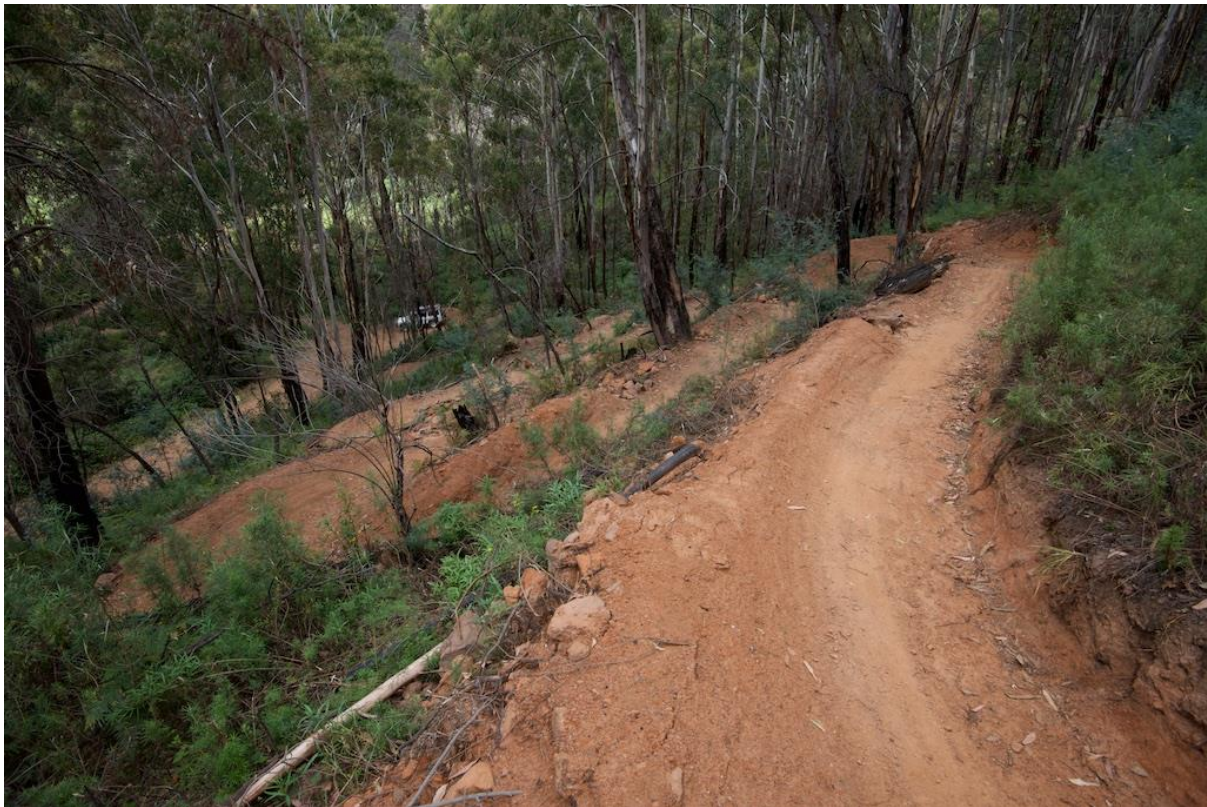
Figure 10 New climbing track, Glenwood State Forest (Photo: H. Berndt). Note the vehicle at the bottom of the slope, for scale. These switchbacks effectively change the vegetation, soils and hydrology of a whole slope. High banks on bends allow for higher speed and rider stability, however they must be built up using surrounding soil, further expanding the area of impact.
