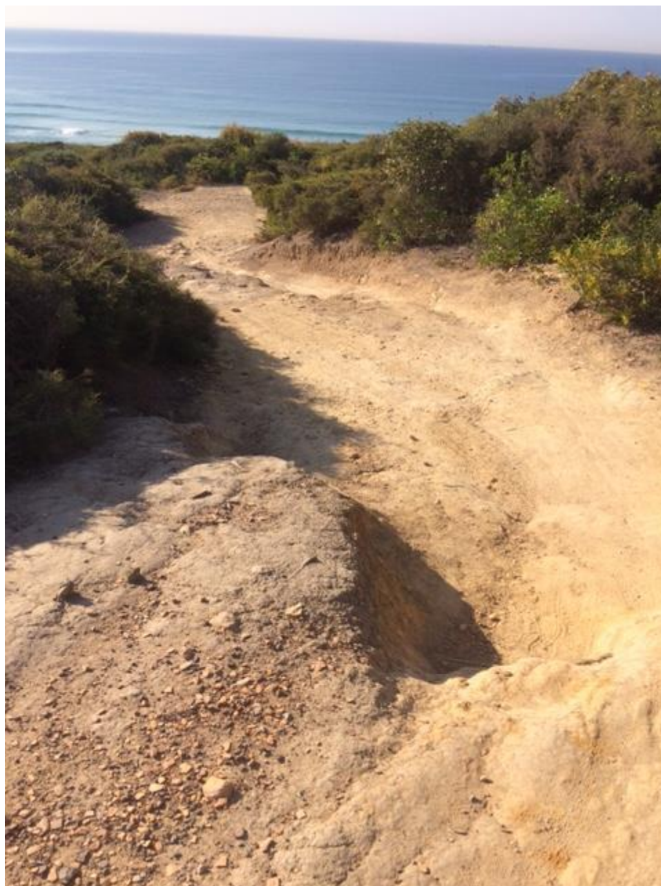
Figure 4 Lateral and vertical soil erosion on mountain bike track, Glenrock SCA (photo: A. Harte). A dedicated single track here has been widened as a consequence of the combination of vulnerable heathland soils and track diversions. This area is not adequately maintained and is actively eroding.
