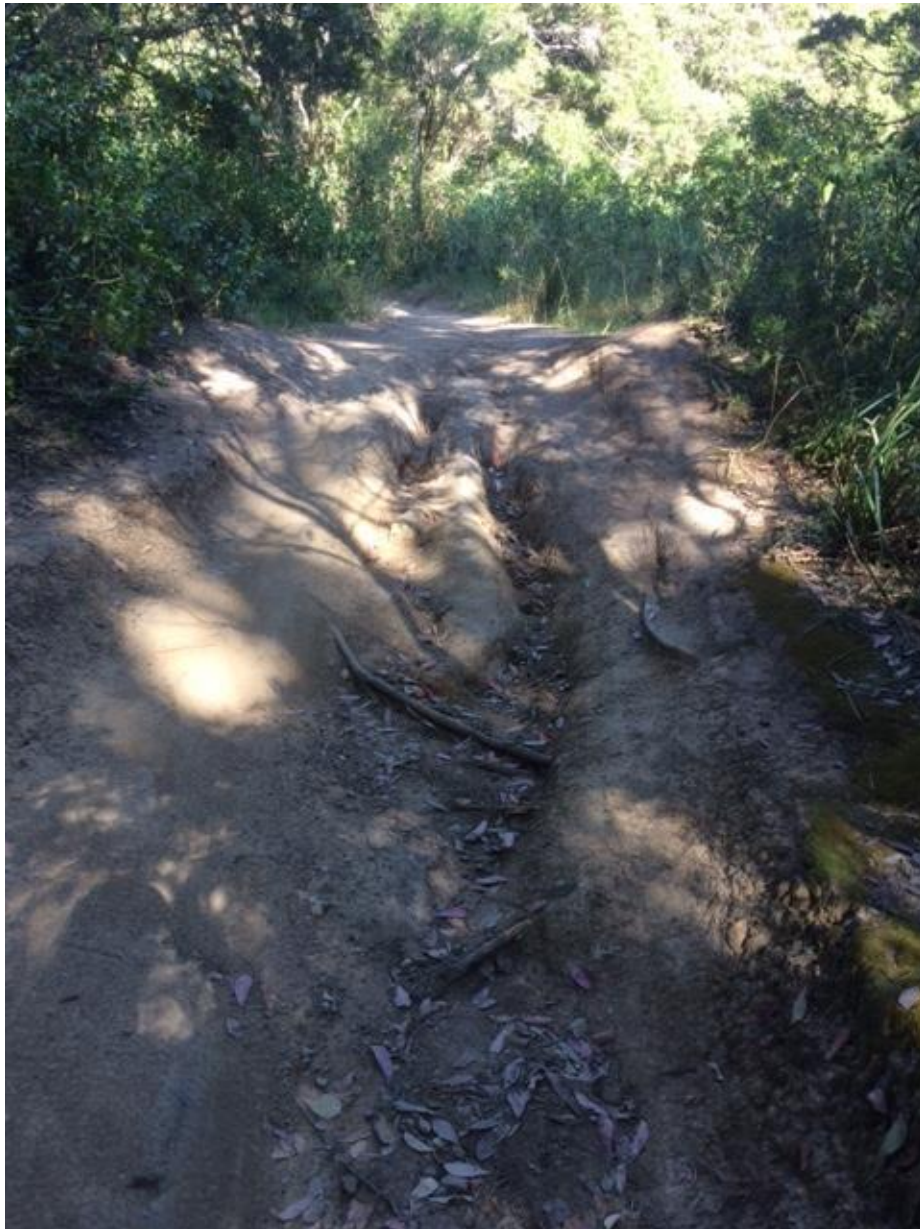
Figure 1 Soil erosion along mountain bike track, Glenrock SCA (Photo: A. Harte). Note the widened track due to diversion around the central rill.
