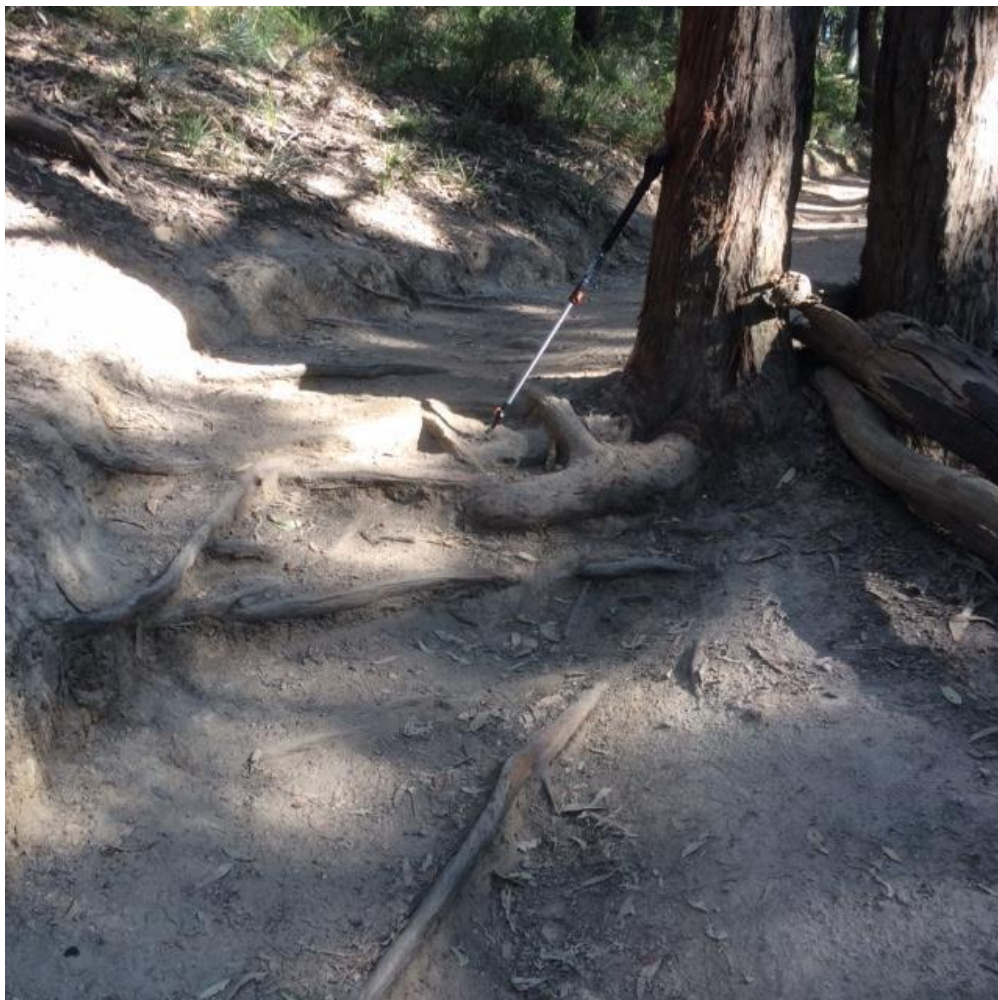
Figure 5 Eroded single track, Glenrock SCA (Photo: A. Harte). Note the deep and wide track and exposed roots.
