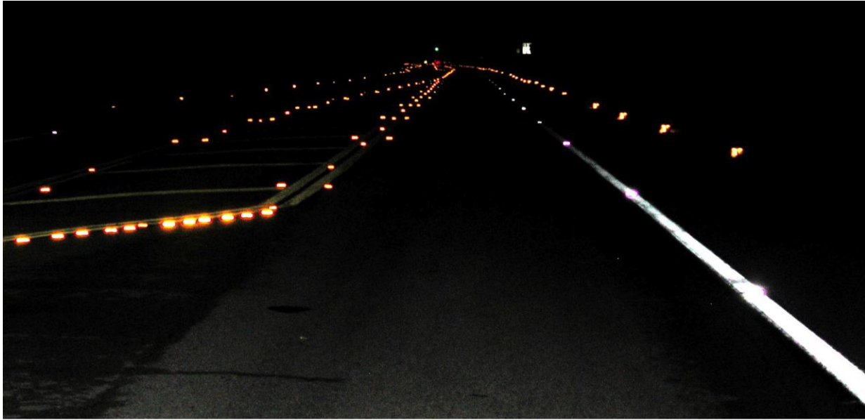
Figure 27. Embedded roadway lighting. These LED lights installed in the pavement are not visible to sea turtles nesting on the adjacent beach and are well received by motorists and pedestrians (Bertolotti and Salmon 2005). Photograph courtesy of Michael Salmon.
